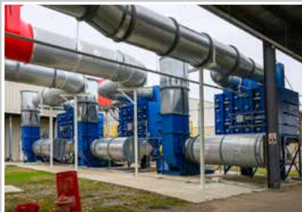
DONALDSON TORIT Downflo Evolution Dust Collectors
