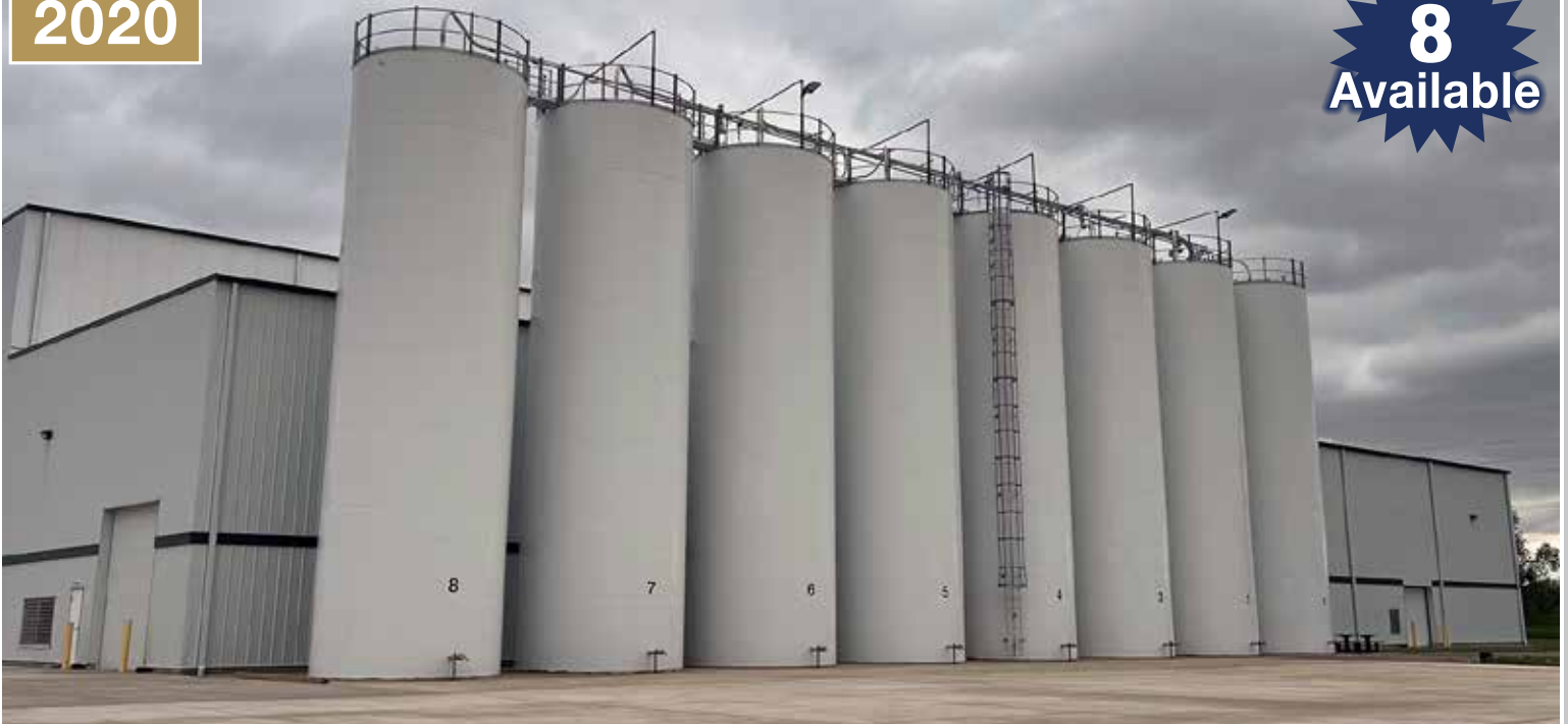
CST Storage Silos
